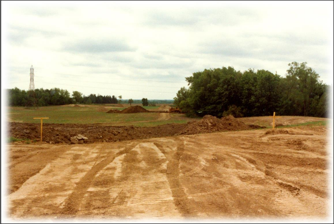
Constructing the new nine
